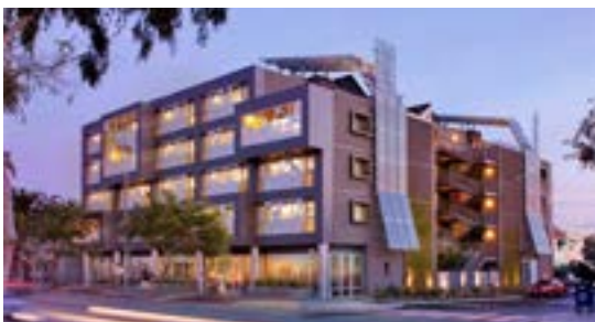
SIERRA BONITA AFFORDABLE HOUSING IN WEST HOLLYWOOD
